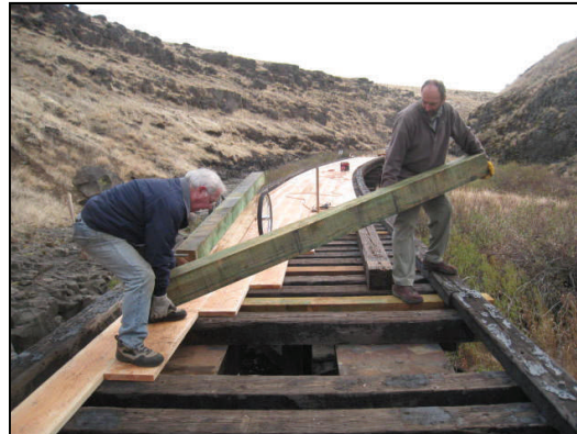
Replacing decaying ties
