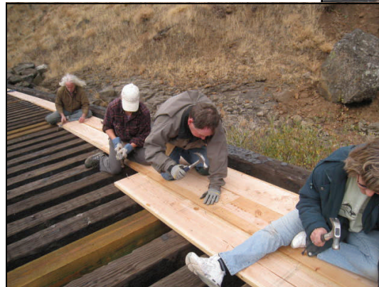
Replacing decaying ties
